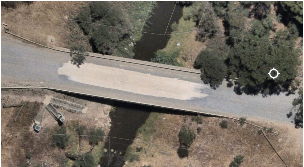
Figure 3 – Cardinia Creek Bridge between McCormack's Road and Chasemore Road
