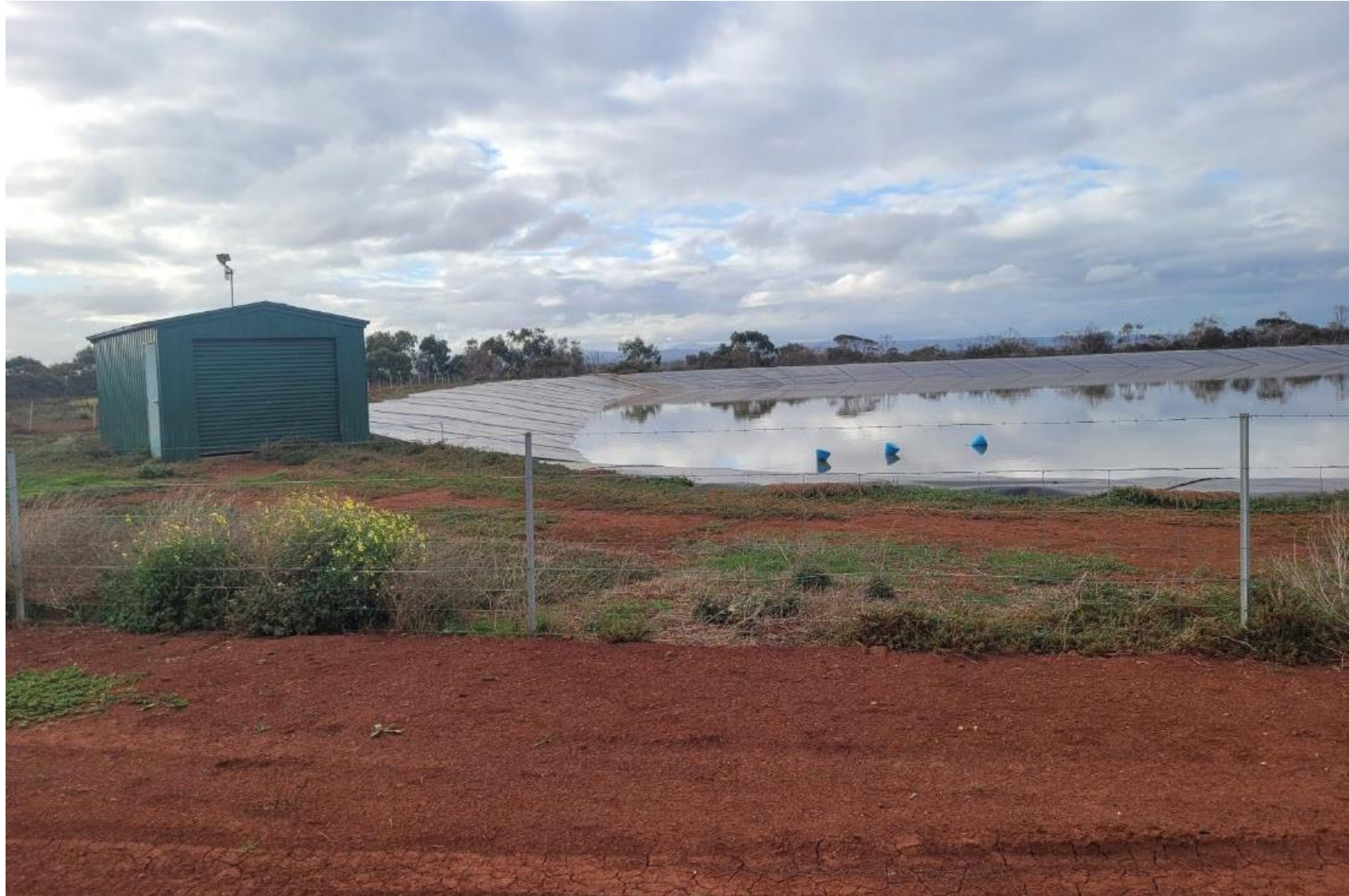
Photo 35 Property parcel 90 (EHP parcel 63) (north-east extent, facing north). Large plastic-lined constructed dam and surrounding soil disturbance in corner of property.
