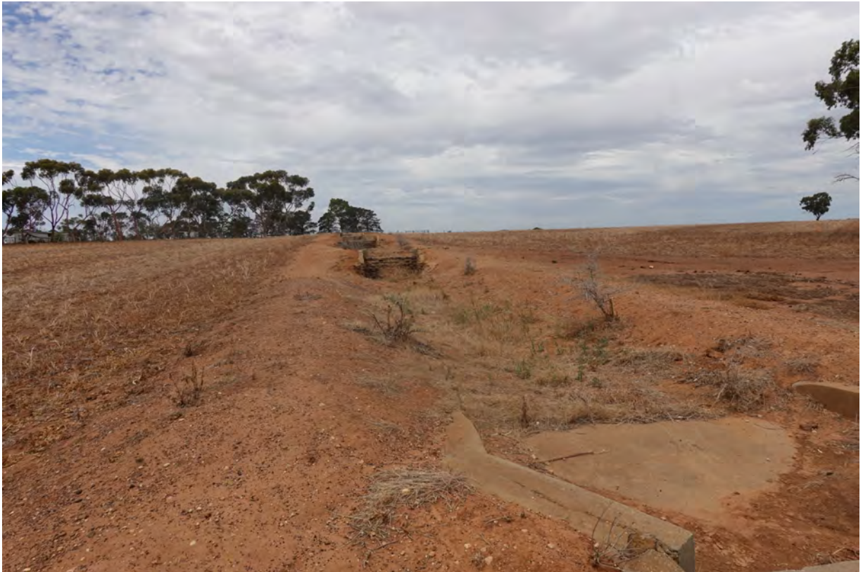
Figure 15. Broad view of the stepped stormwater drain on the south side of the Kerr Farmhouse driveway, near its intersection with Smiths Road, showing the sequence of drop structures stepping down-slope. (Source: Touring the Past, 4 February 2026)
