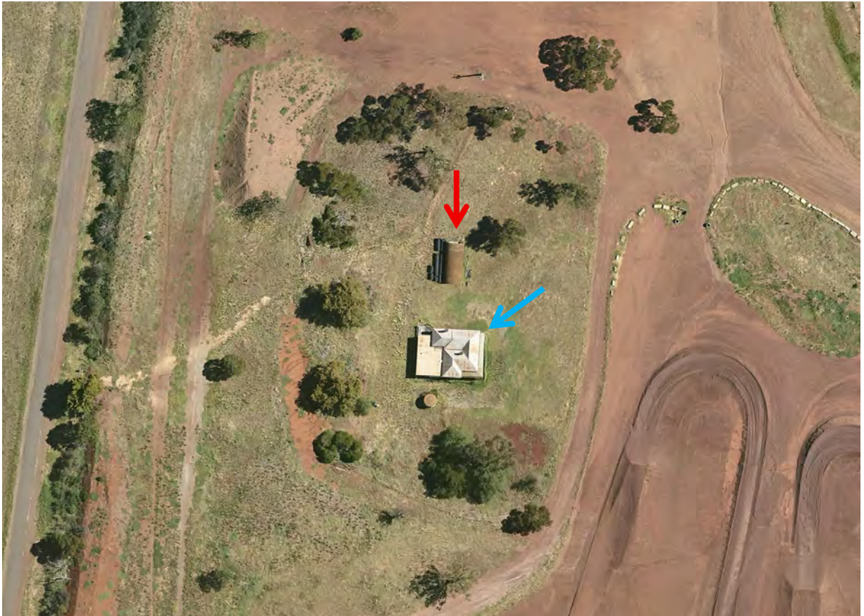
Figure 11. Aerial image of Montrose (blue arrow) and Nissen Hut (red arrow). North is top of image. (Source: Metromap, January 2026)
