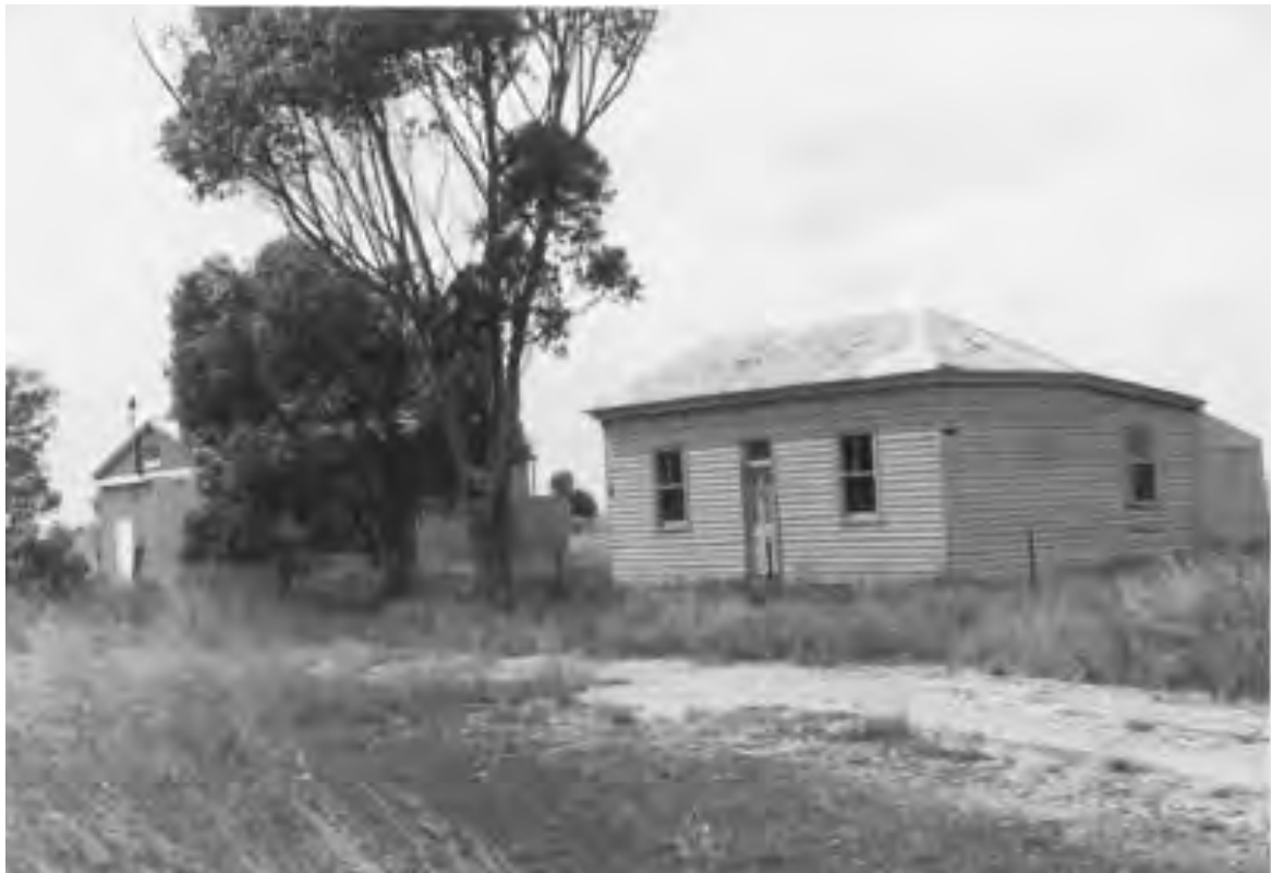
Figure 1. Parwan Post Office, operated 1901-87, location unresearched, building no longer extant. (Source: National Archives of Australia, B5919)
