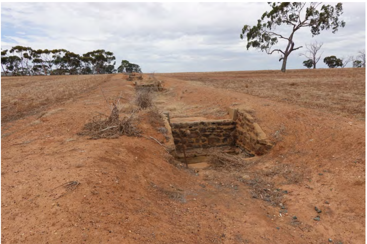
Figure 16. Detail of one of the stepped 'drop' structures within the stormwater drain, showing rubble stone masonry sidewalls with concrete wing walls and apron. (Source: Touring the Past, 4 February 2026)
