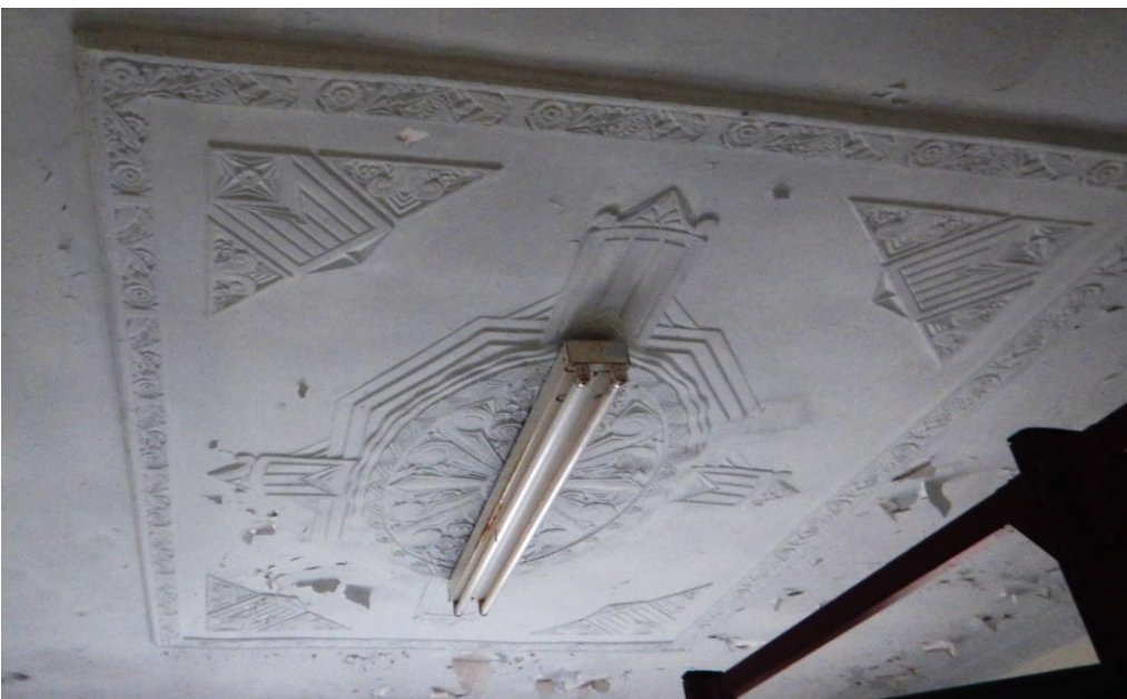
Figure 44 Art Deco ceiling rose in the homestead (G. Vines 26/3/2026)
