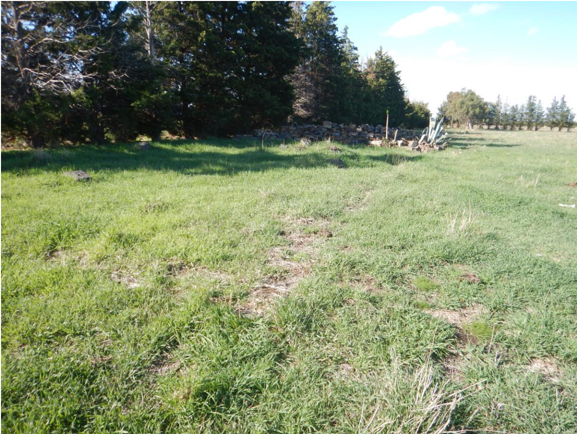
Figure 26 Bleak House Ruin showing foundations in foreground looking north (G. Vines 26/3/2026)
