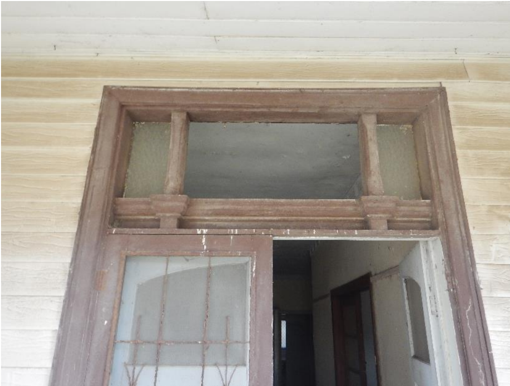
Figure 45 Detail of headlight above main entrance showing timber details (G. Vines 26/3/2026)
