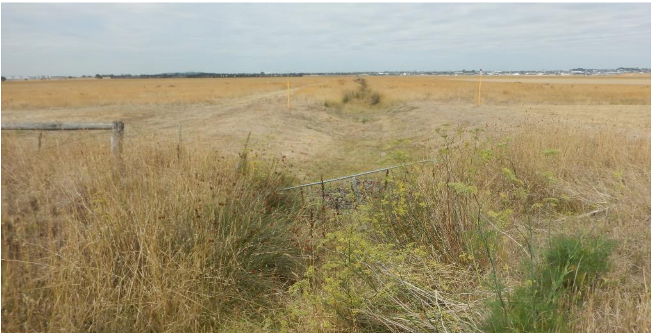
Figure 20 Typical north-south drain in the study area looking south from Gunns Gully Road (G. Vines 26/2/26).
