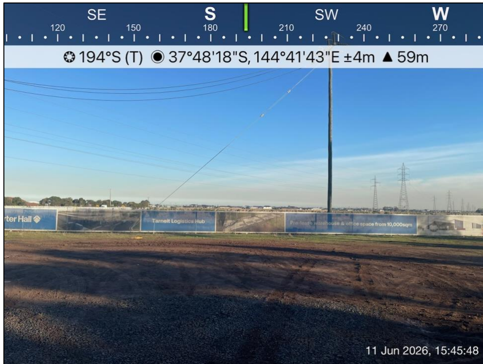
Figure 11 – Land cleared for development, south-west of the corner of Boundary Road and Derrimut Road.
