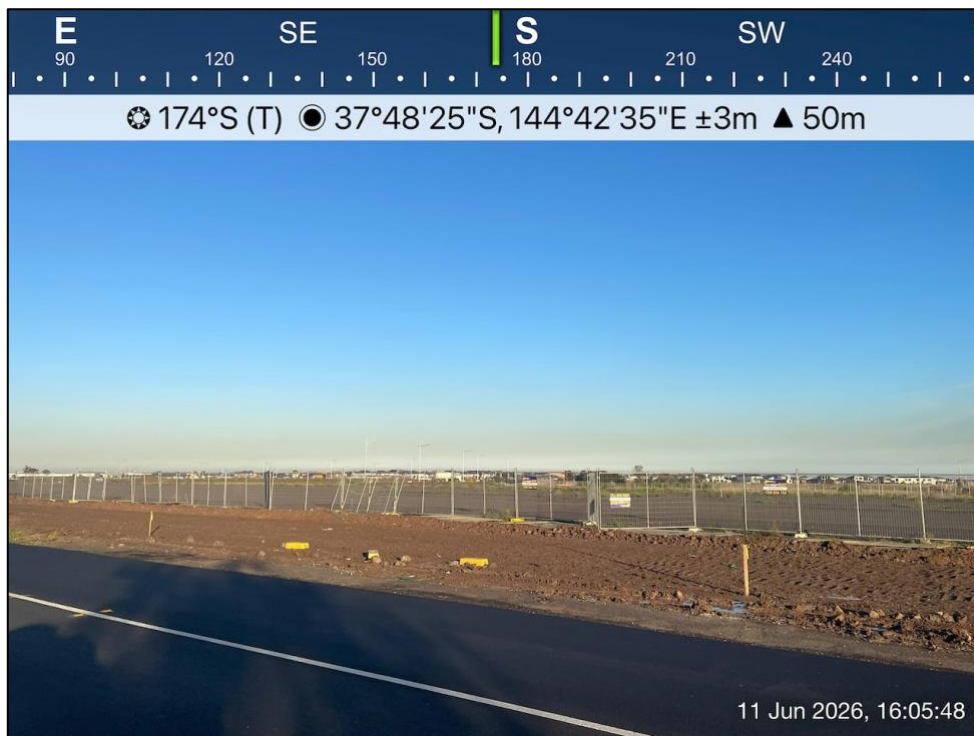
Figure 12 – Land cleared for development, south of Boundary Road.
