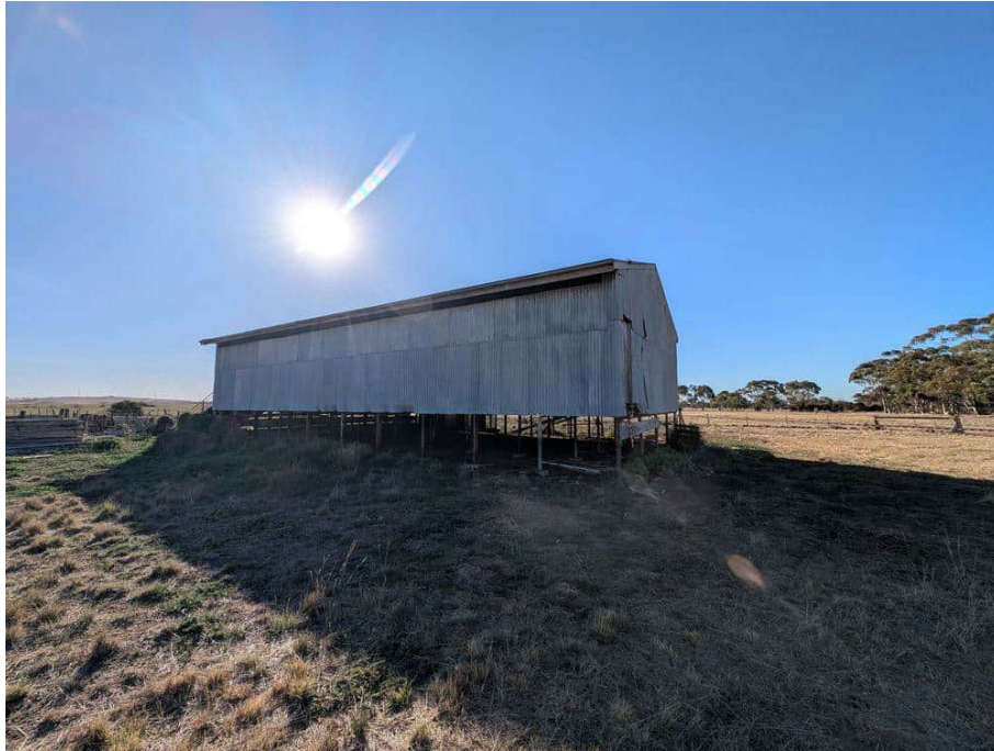
Photograph 11: Site Walkover - Parcel 3 (E) – 2
