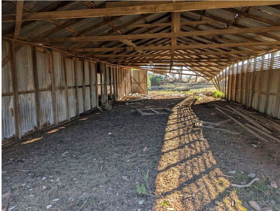
Photograph 7: Site Walkover - Parcel 3 (SE) - 2
