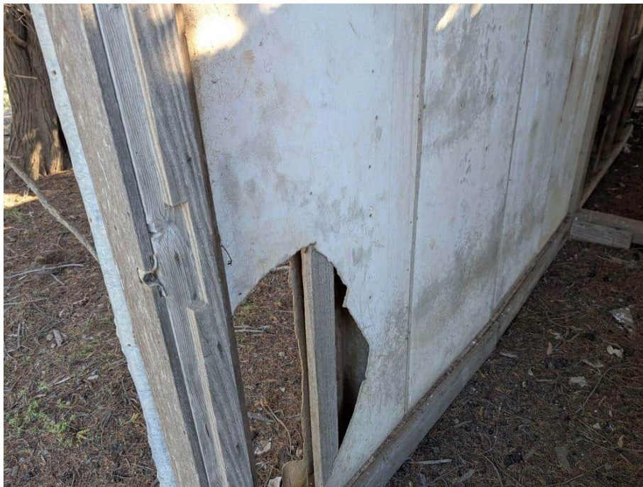
Photograph 8: Site Walkover - Parcel 3 (SE) - 2
