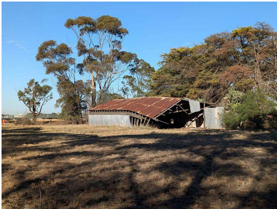
Photograph 6: Site Walkover - Parcel 3 (SE) - 2
